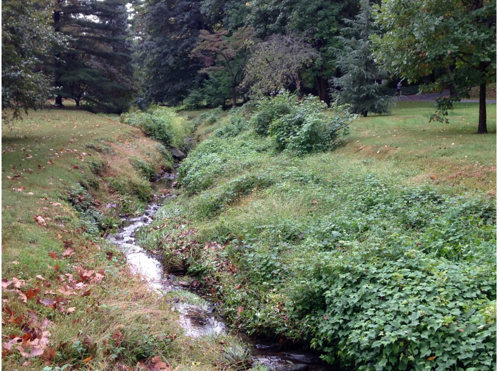
Scoured and eroded banks Invasive species flourish
