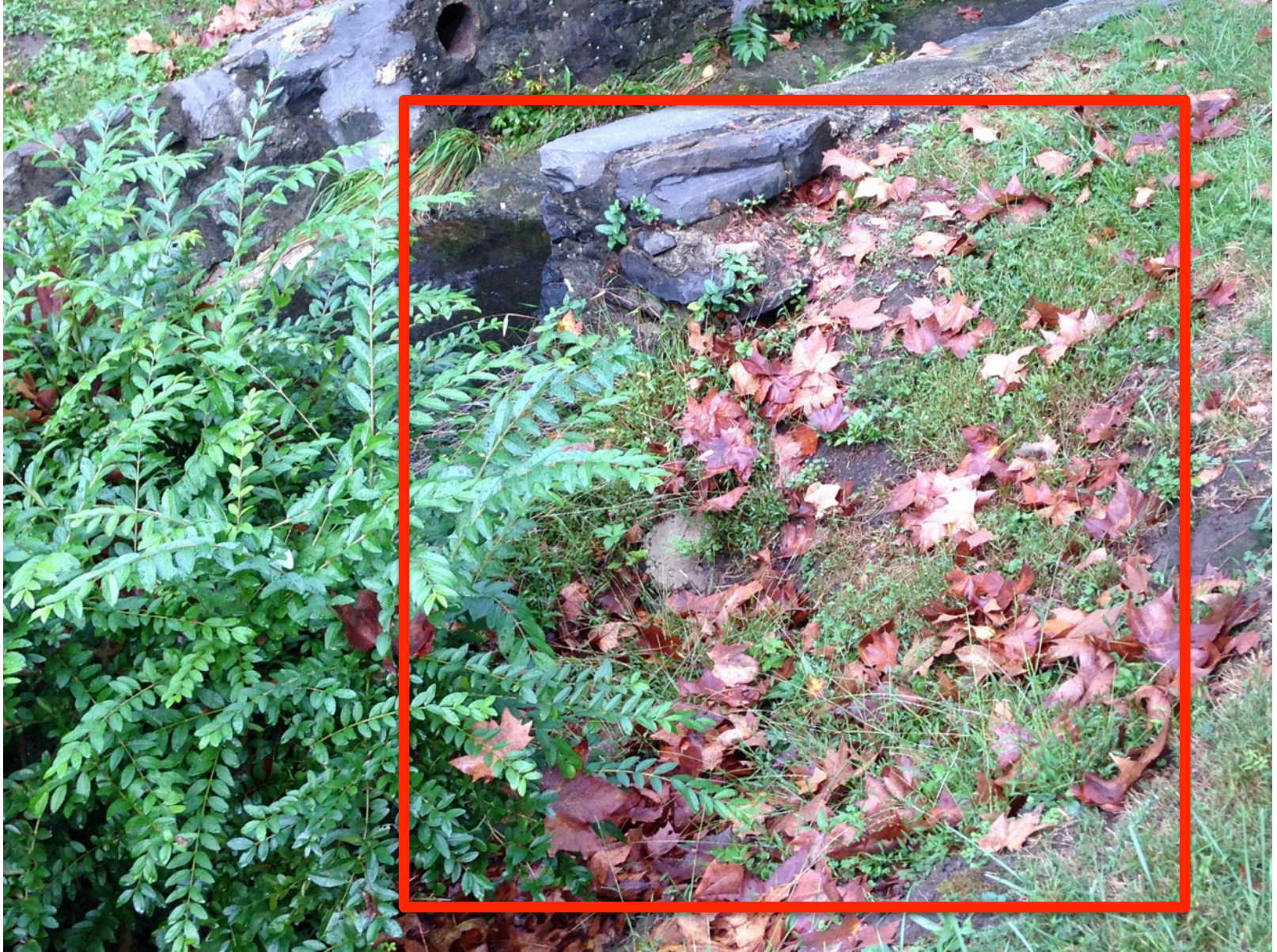
Eroded bank at end of channel wall
