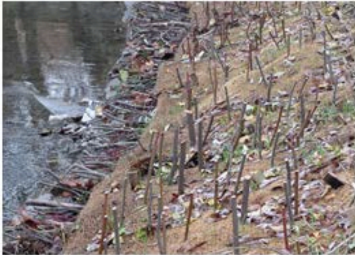
Live stakes and brush mattresses installed in a stream bank stabilization site
