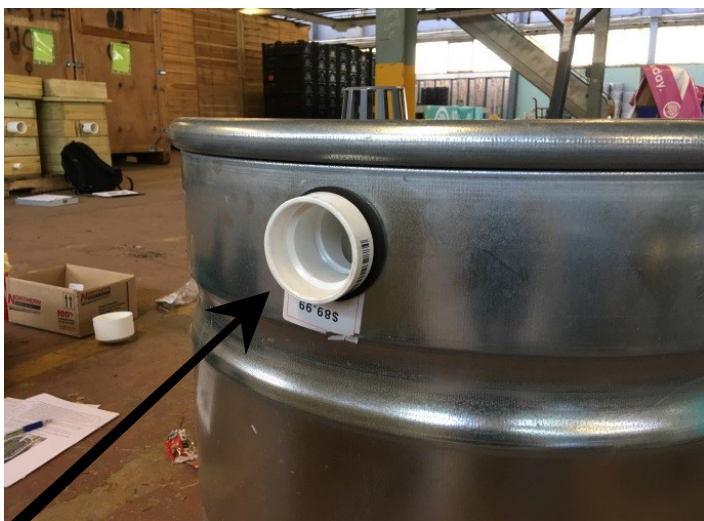
Figure 5b. Overflow riser installed with atrium grate
