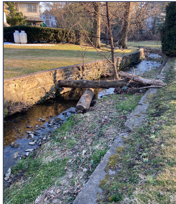
The East Branch of Indian Creek is channelized through 3 Elmwood, and its riparian buffer is non-existent.
