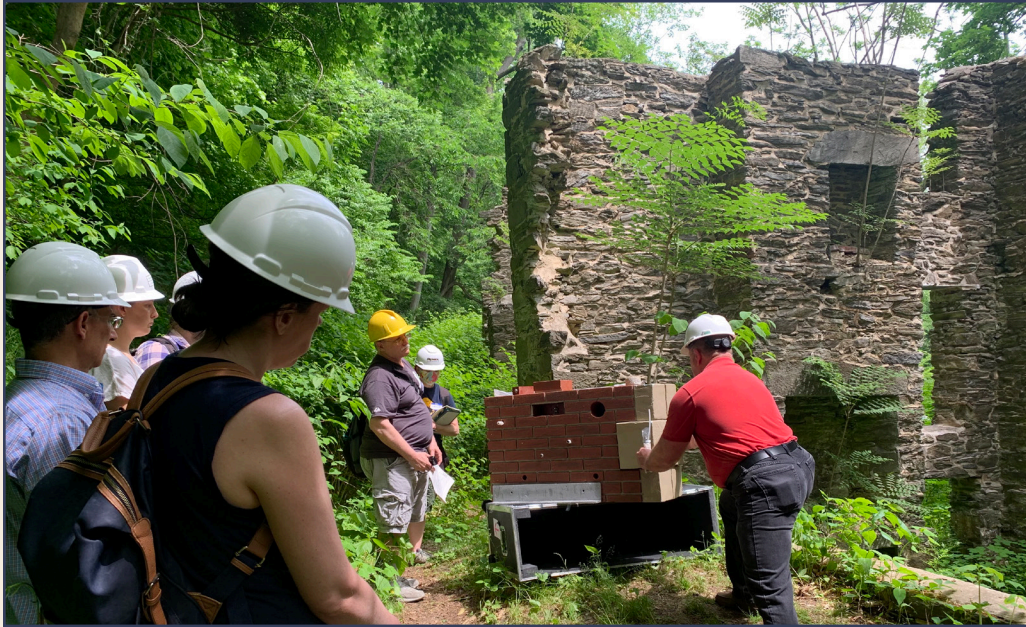
Preservation professionals demonstrating mortar repair on historic tenement buildings.
