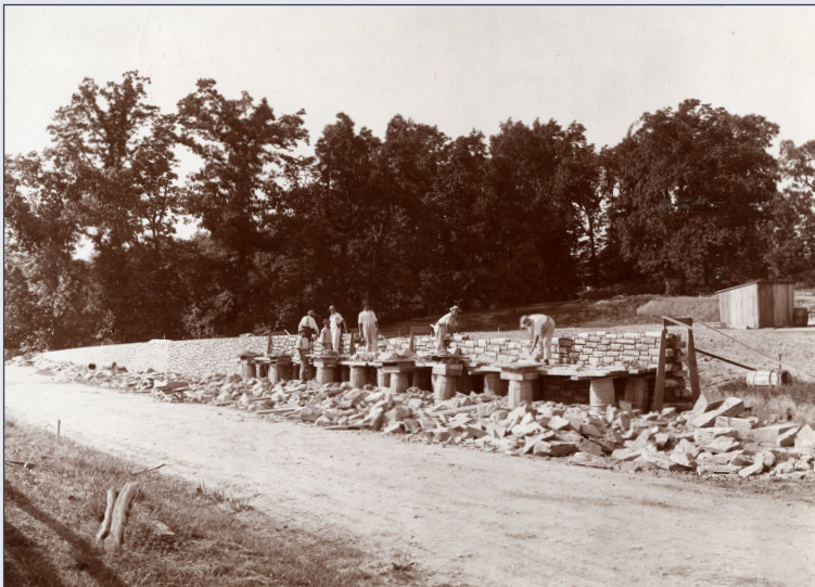
Masons building the wall along Percival Roberts’s Pennhurst estate.
