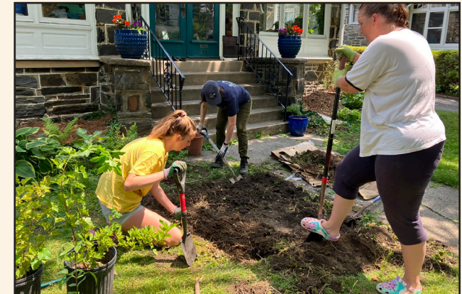
The Conservancy digs a rain garden to capture roof runoff in Narberth.
