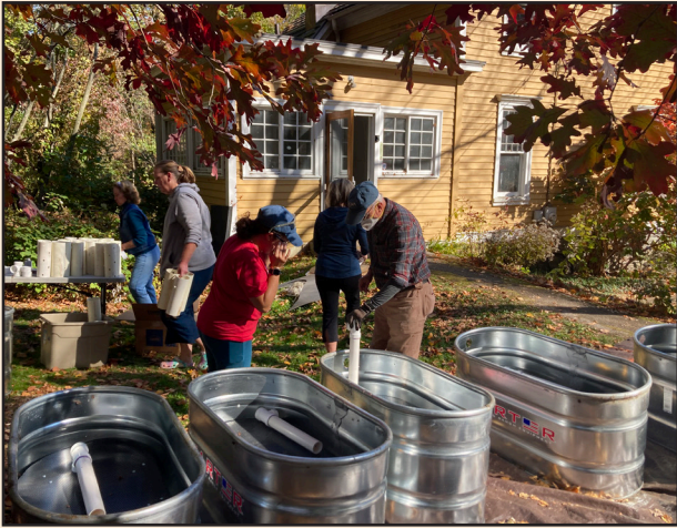
Partners across organizations come together to work on downspout planter construction.
