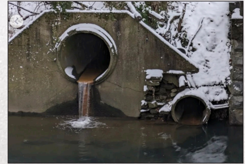
Runoff from salt-treated roadways flows into storm drains, then directly into Cobbs Creek.
