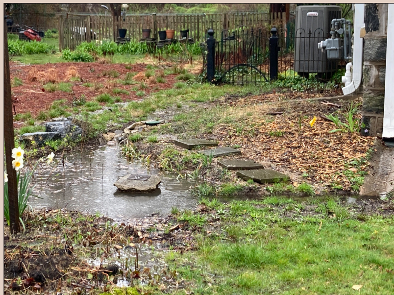
A rain garden in Narberth effectively retains a significant amount of rainfall during spring storms. Take note how downspouts channel roof runoff directly into the garden.
