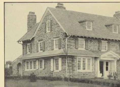
The shingled roof sheltering the first-story windows is a feature commonly called the "Germantown hood"
