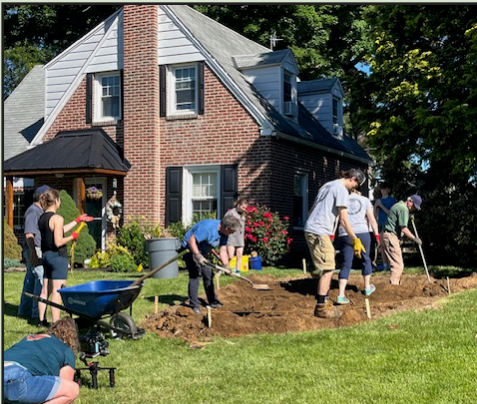
Lawn removal can be done manually with shovels and hand tools.
