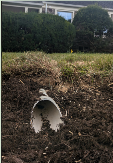
A gutter pipe diverts rain from a roof, reducing the amount of water that reaches the storm sewer system.
