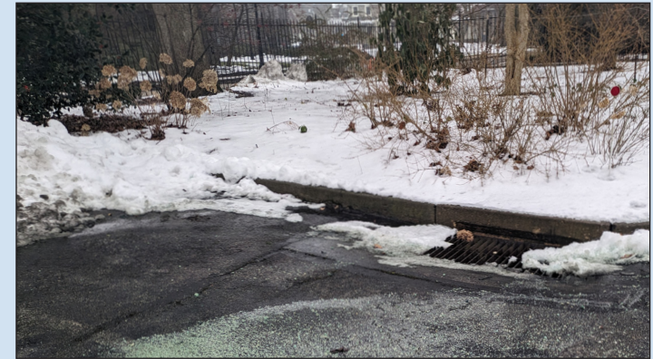
An all too familiar scene - excessive salt on a parking lot, directly next to a storm drain.
