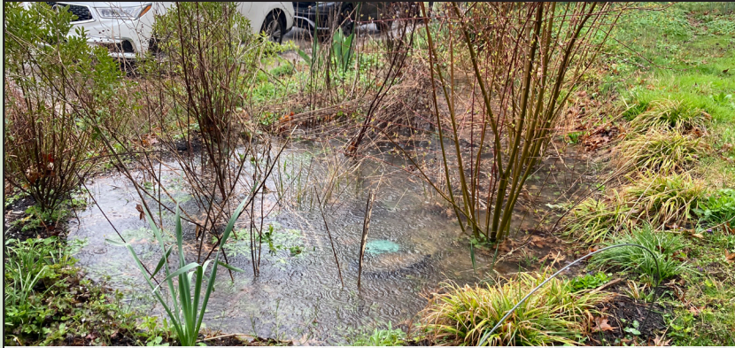
The basin shape of a rain garden forces rain to seep into the ground, keeping it out the storm sewer that leads to a creek.
