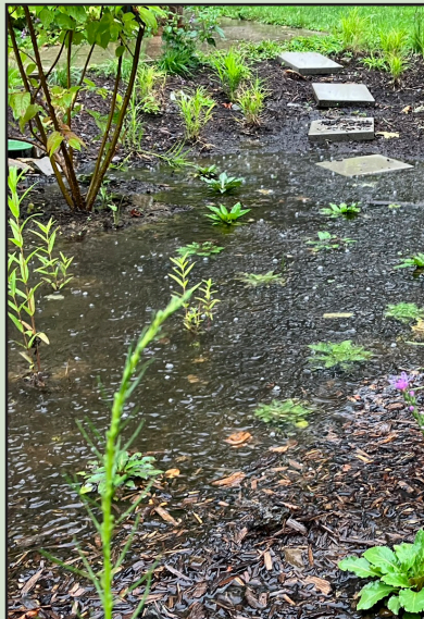
GGC rain garden during a storm. The garden captures runoff from the roof and from the lawn.
